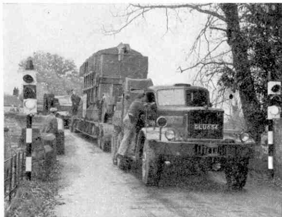
Anxious moments at Stopham's 14th century bridge as a heavy tractor and trailer carrying a giant 95-ton Transformer passes over it on its way to Fontwell, Sussex. Photograph by G. G. Garland.
