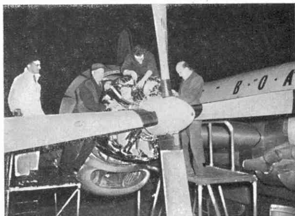
The servicing of aircraft goes on throughout the 24 hours at London Airport. Here the night duty engineers are seen working on a B.O.A.C. Stratocruiser. Photograph by courtesy of British Overseas Airways Corporation.
