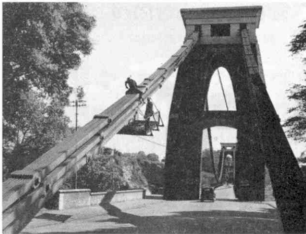
A never-ending task. As soon as painters have taken their cradle from one end to the other it is time to begin all over again.
