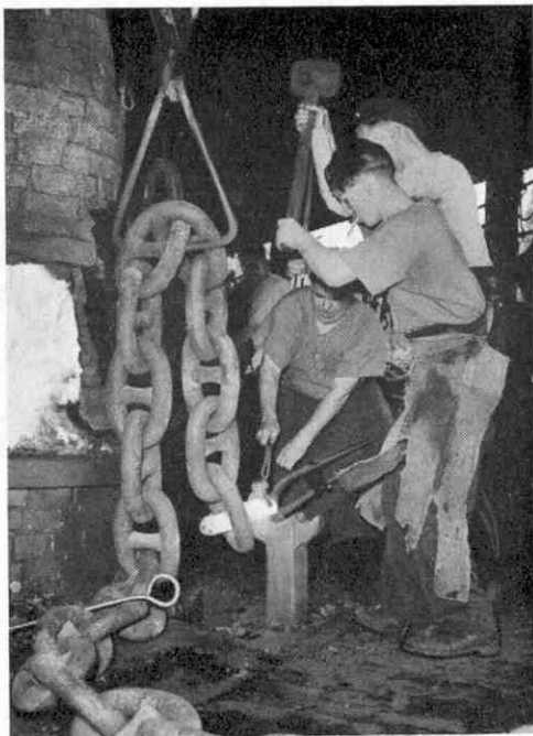
Hand welding side-welded chain cable with the heavy two handed hammer known as the Johnny. This illustration and the photograph on which our cover is based are by W. K. V. Gale.
