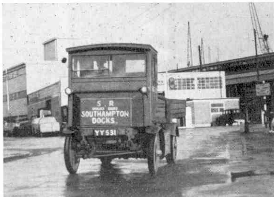
A veteran lorry that began work at Southampton Docks in 1922. It is electric, with chain drive, and was supplied by Richard Garratt and Son, Suffolk. Up to the end of 1952 it was often seen on the roads in and around the Docks, but was then withdrawn from service on public roads. Photograph by H. Meyer, Chandler's Ford.
