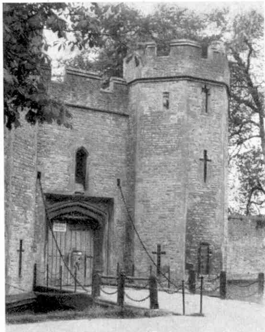
This gateway at the Bishop's Palace at Wells, Somerset, provides a notable example of a drawbridge of the later Middle Ages.
