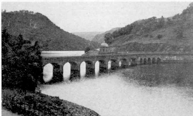
The road over the Careg Dhu Dam, in the Elan Valley, Central Wales. Photograph by R. Bruce, Ashtead.
