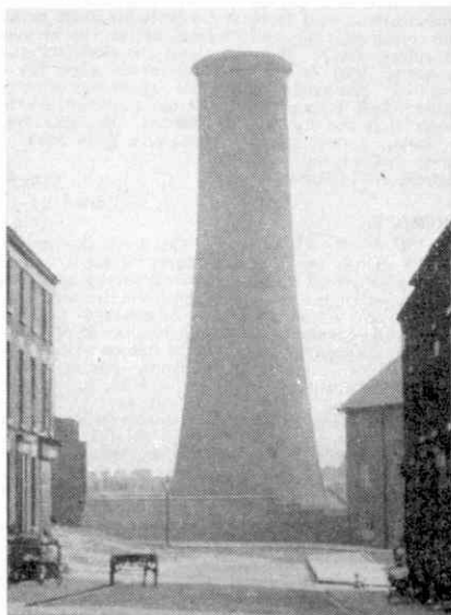
This giant chimney, to be seen in Liverpool alongside the L.M.R. line from Lime Street Station to Edge Hill, was built in 1870 as part of the system of ventilating the long tunnel through which the line then ran.
