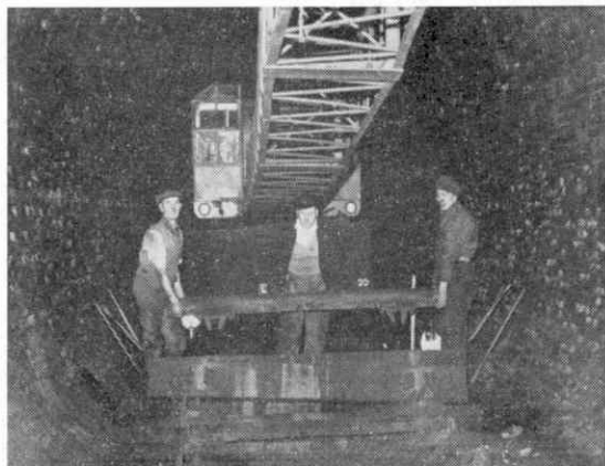
Lifting track in Tyler Hill Tunnel.
