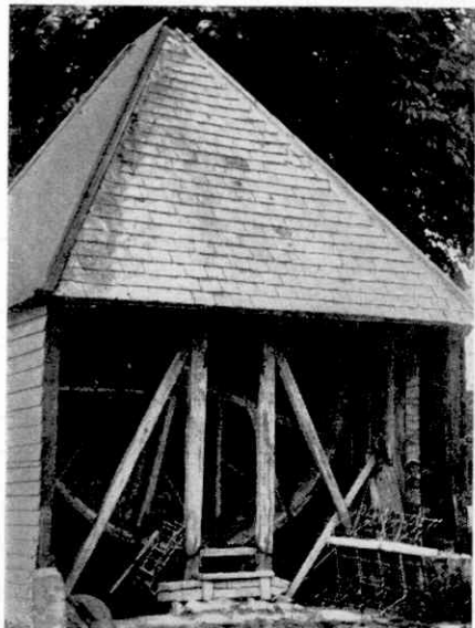
The donkey wheel at Saddlescombe farm, which pumped water until comparatively recently. Photograph by A. Phillip, Hassocks.
