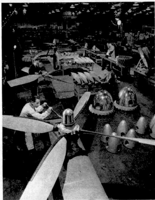
De Havilland variable pitch propellers in production. In the foreground a 4-bladed propeller is being assembled. Photograph by courtesy of de Havilland Enterprise.
