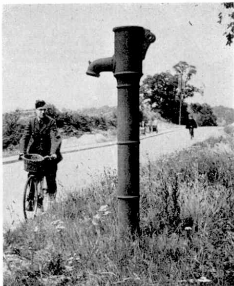
Not a village pump, but one erected to provide water for keeping down dust on turnpike roads in coaching days. It is near Hartley Witney, Hampshire. Photograph by Reece Winstone.
