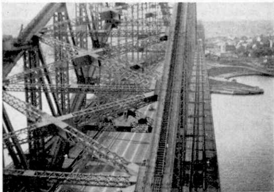
The view in the opposite direction, from the Pylon Lookout, showing the steelwork of the giant arch of the bridge.
