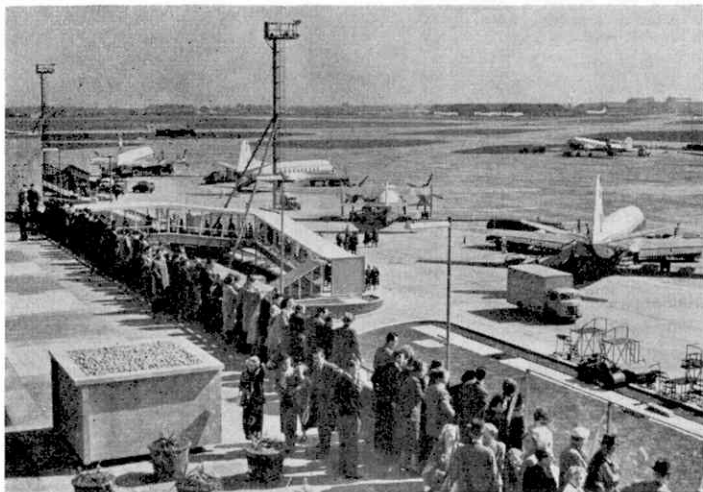
This view of London Airport shows one of the L-shaped ramps by which passengers pass directly to and from their aircraft. British European Airways photograph.
