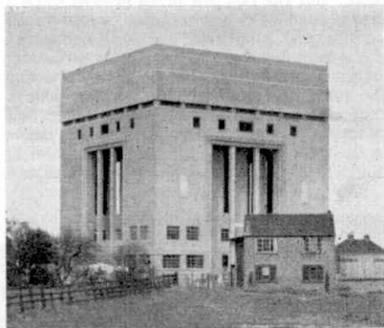
This water tower at Spalding is the largest of its kind in Britain. Photograph by R. Dixon, Spalding.
