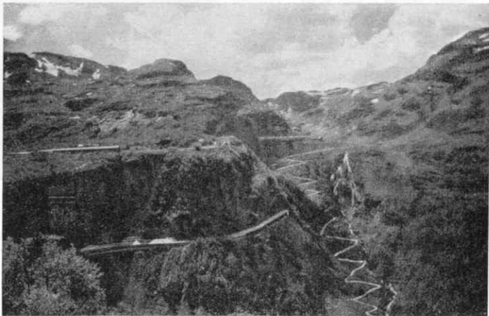
Three levels of the Flam Railway. This climbs nearly 3,000 feet in its course of 12 miles, in which it tunnels in vast loops in the mountain side. On the right are the zig-zags of the road.
