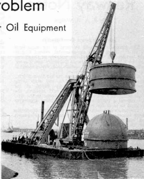
Our two illustrations show parts of a catalyst hopper on a floating crane on Tees-side, and one of the parts being lowered on to the deck of the vessel in which they travelled to South America. Shell photographs.
