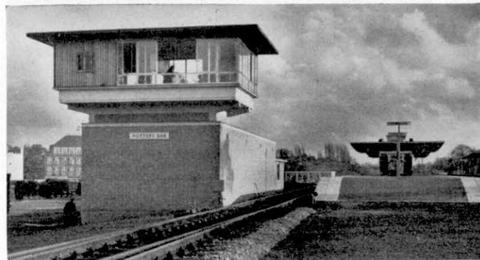
The signal box and north end of the new Potters Bar Station B.R. Eastern Region.
