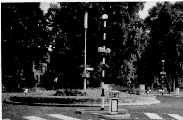
A new type of street lamp at Dulwich. Within its cylindrical lantern are 5 G.E.C. cold cathode fluorescent tubes. Photograph by M. F. T. Fife, Dulwich.
