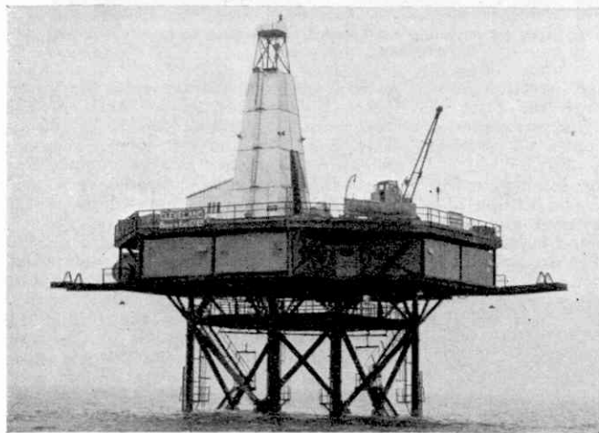
In this picture the National Coal Board's experimental drilling tower is seen set down on the sea bed, with drilling in progress.
