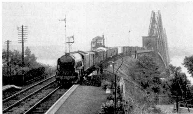
Looking at the Forth Bridge from Dalmeny Station. The camera of J. D. Pawley has caught an approaching fast freight train in charge of a Pacific.
