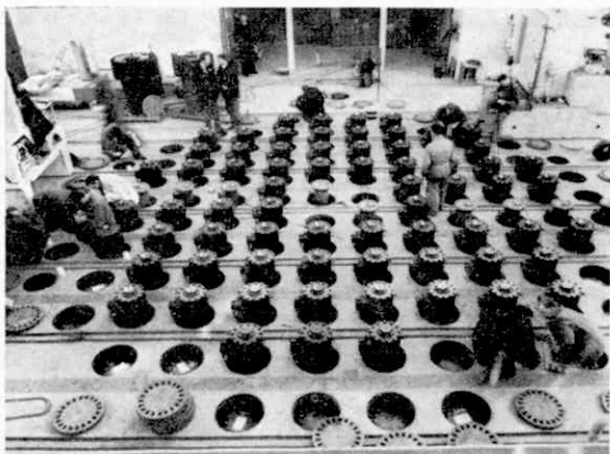
This picture shows preparations being made to insert uranium rods at the top of the first of two piles at the Calder Hall atomic power station. The first of these piles has now started working.
