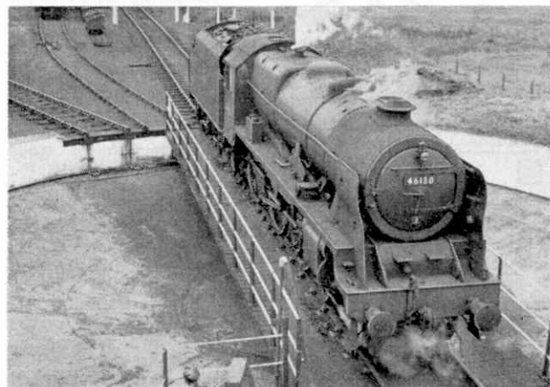
This real turntable, at Holyhead, has several shed tracks radiating from the turntable itself. Photograph by G. Clarke.
