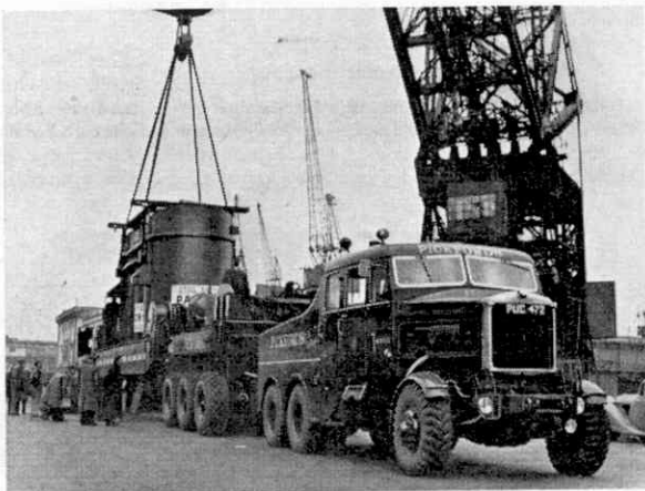
The transformer lowered on to the carrier on which it travelled by road to Ferrybridge.
