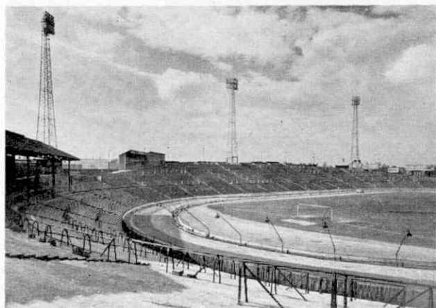
Tall floodlighting towers in the Chelsea Football Club's ground at Stamford Bridge. Photograph by courtesy of the General Electric Co. Ltd.
