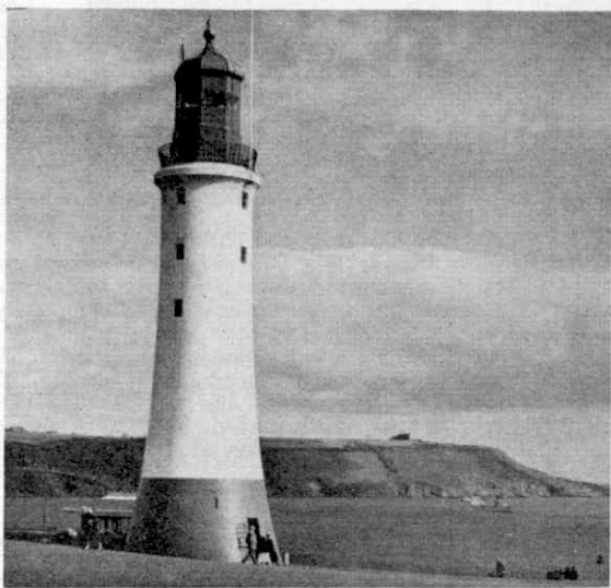
The upper part of Smeaton's Eddystone Rock lighthouse now stands on Plymouth Hoe, and is seen in this picture. The stump is still to be seen on the rock, a monument to the great engineer who built this famous lighthouse. Photograph by F. Bunce.
