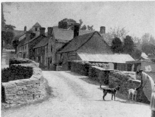
Clun Bridge, Shropshire, which has deep recesses in its walls. Photograph by A. Phillip, Hassocks.
