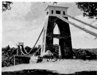
Clifton Suspension Bridge, Bristol
