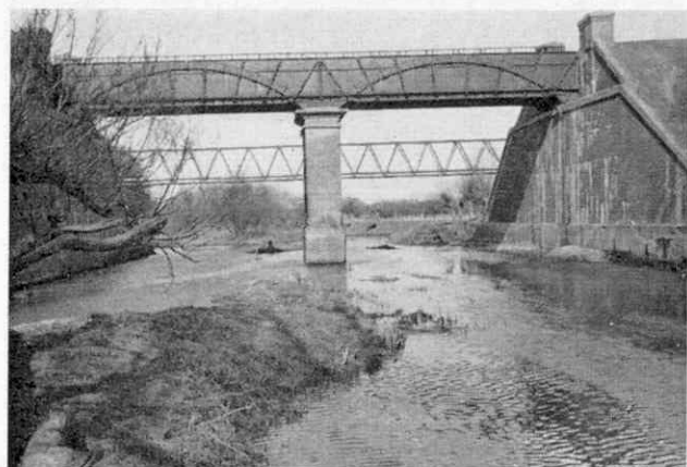
The aqueduct carrying the Grand Union Canal across the River Ouse at Wolverton.
