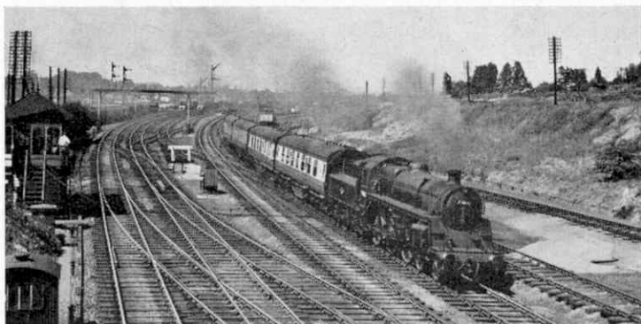
A fine length of four-track railway near Kettering, including a double junction, crossover roads and crossings. Photograph by P. J. Lynch.
