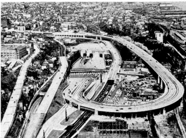
An aerial view of the approaches and connections to the Lincoln Tunnel on the New Jersey side.
