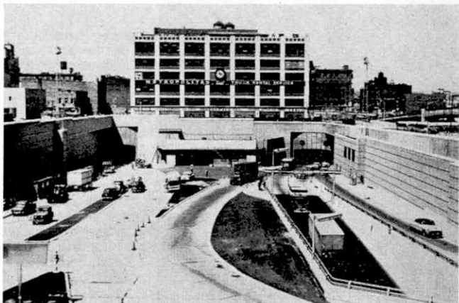
The New York exit portal of the recently completed third tube of the Lincoln Tunnel is seen on the left in this picture. The portal of what is now the central tube of the three is on the right.
