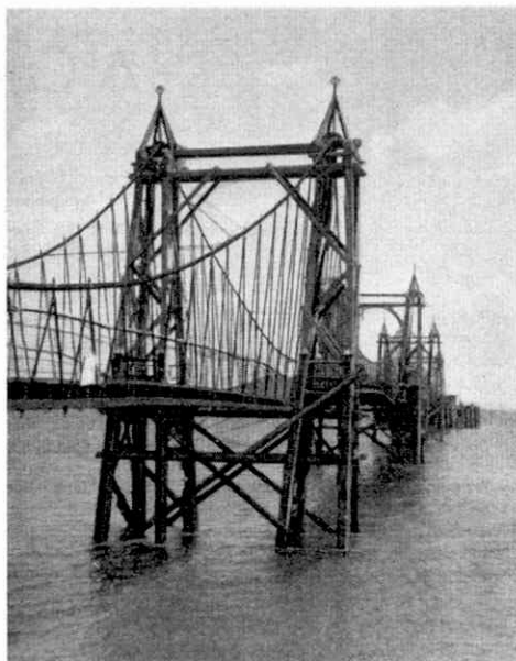
The unusual wooden pier that was formerly to be seen at Seaview, Isle of Wight. This photograph and the accompanying notes are by P. Norris, Ryde.
