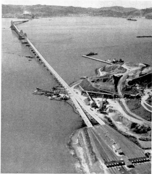
The bridge from Richmond to San Rafael stretches across the northern part of San Francisco Bay. It is 21,343 ft. in length, and in this respect is exceeded only by the San Francisco-Oakland Bay bridge, which is 1,377 ft. longer. The Richmond-San Rafael Bridge is roughly 3\frac{1}{2} times as long as the Forth Bridge and 13 times as long as the great bridge across Sydney Harbour, in Australia.
