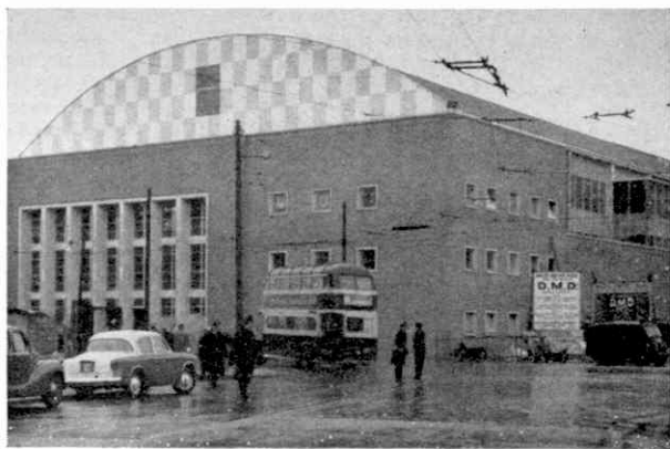
The Empire Swimming Pool, Cardiff, nearing completion. Here the swimming and diving events of the 1958 Empire Games will take place.
