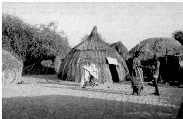
A compound on the shores of Lake Chad. The houses are of straw on stick frames, as mud for building is very scarce here.
