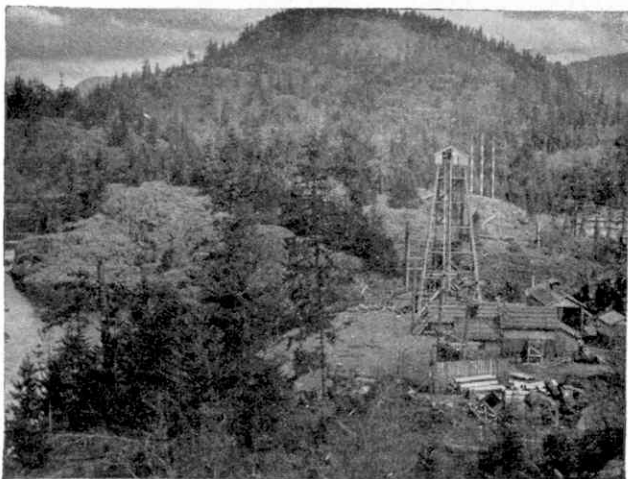
The vertical shaft from the installation in this picture descends 572 ft., and from the bottom a 300 ft. tunnel leads to a maze of galleries packed with explosives inside Ripple Rocks, an underwater mountain in the waterway between Vancouver Island and the mainland of Canada that was eventually blown to pieces. Illustrations from photographs by the author.
