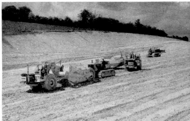
Tractors and scrapers grading a section of the new Motorway.
