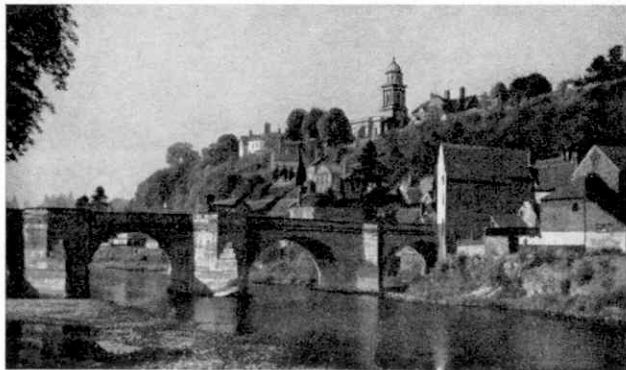
The view from "Foundry Yard", today. Telford's Doric Tower in Hightown overlooks the Severn and the Bridge.
