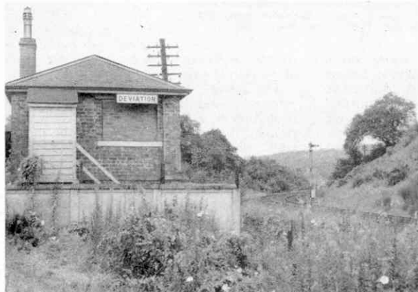
"Deviation" signal-box, Grosmont, where the new line constructed in 1847 branches off the original one (1836).
