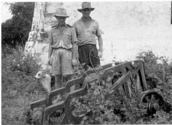
The old signal gun carriage at Khijiri.
