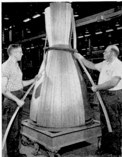
Building up a tubular construction combustion chamber for rockets. The tubes are brazed together after assembly.
