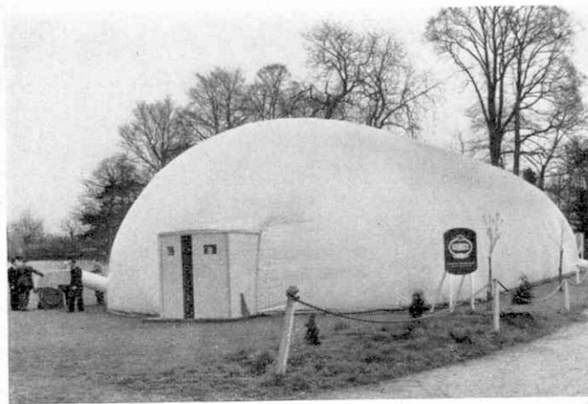
The portable "building" seen on the left is just blown up to erect it.
