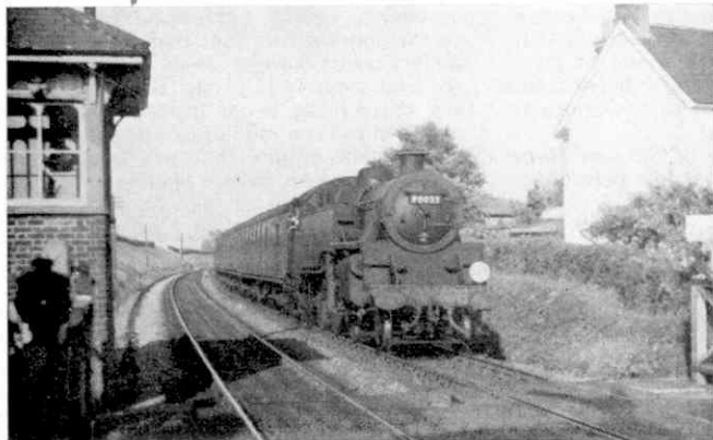
B.R. Standard 2-6-4 Tank No. 80032 with a train from Tonbridge to Brighton. Photograph by J. A. Fleming.
