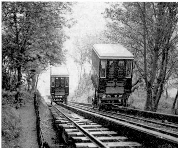
The Babbacombe Cliff tramway, near Torquay, the longest passenger lift of its kind in Britain.
