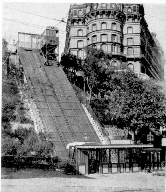
St. Nicholas' Cliff lift, Scarborough, one of four such inclined tramways at this Yorkshire resort. Photographs reproduced by courtesy of J. & E. Hall, Ltd., Dartford.
