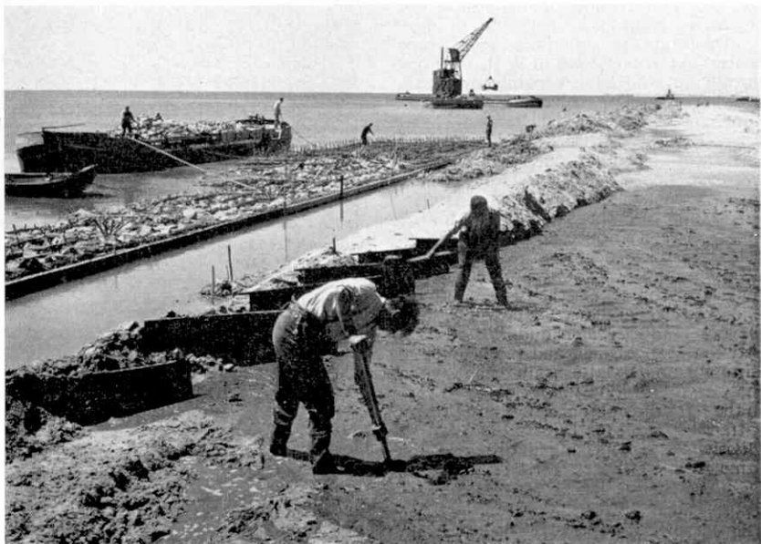
Man's battle to win land and homesteads from the sea—building dykes at East Flevoland.
