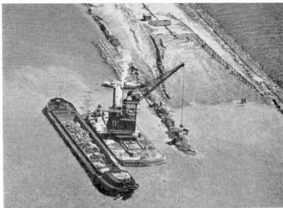
An aerial view of one of the many floating cranes used in the huge reclamation scheme.
