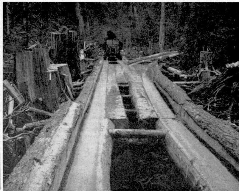
Left: Magnificent timber made possible the world's longest plank road over ground on which no other type of road could be built. Below: Traffic from both directions on the straight "one-way" plank road was made possible by "sidings" within sight of each other. Pictures by courtesy of the British Columbia Forest Service.
