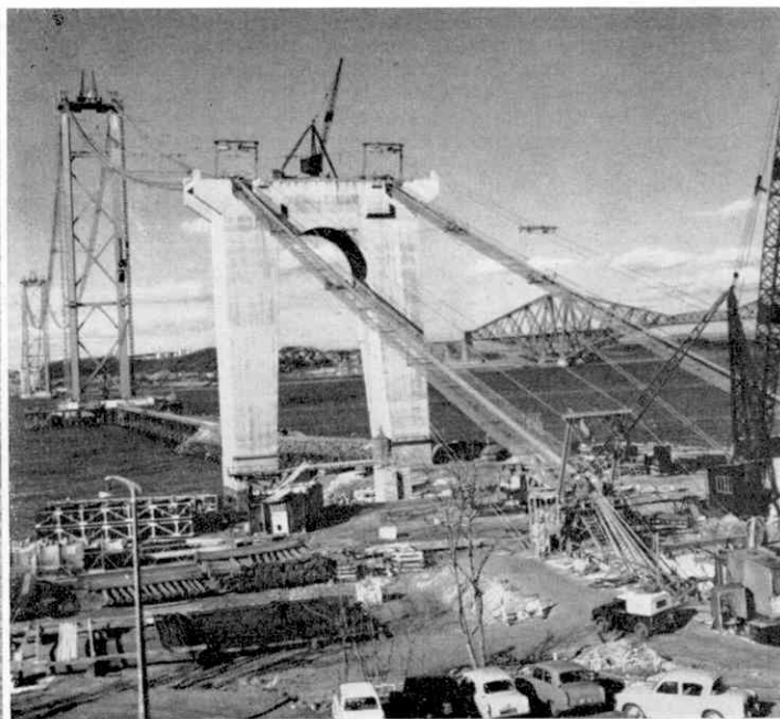
Top: High above Queensferry "spinners" are seen at work tensioning the cables 550 feet up. Left: In this unusual view the men at work on the bridge appear like human flies in the trough of the bridge's enormous span. Below: The business end of the bridge where the suspension cables are anchored, showing the world-famous railway bridge in the background. Pictures by courtesy of Keystone Press Agency Ltd.
