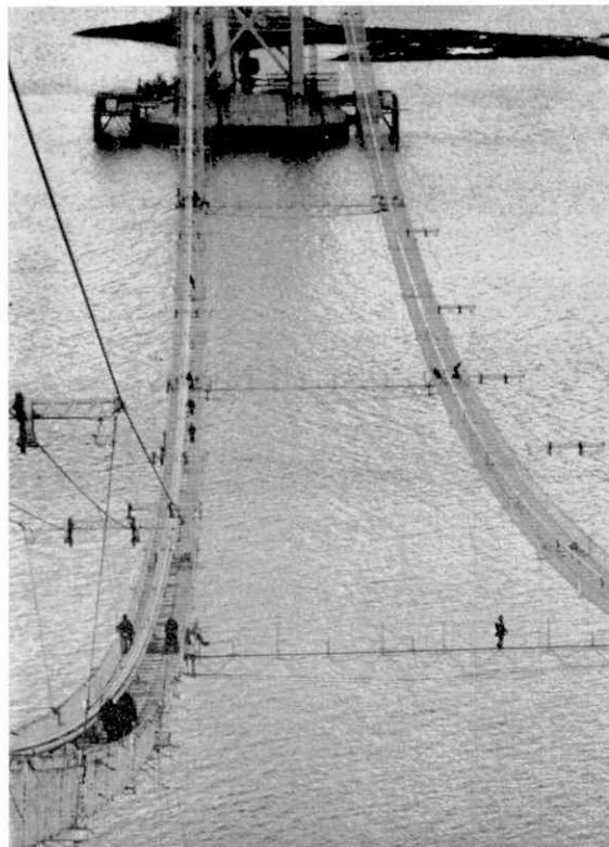
Top: High above Queensferry "spinners" are seen at work tensioning the cables 550 feet up. Left: In this unusual view the men at work on the bridge appear like human flies in the trough of the bridge's enormous span. Below: The business end of the bridge where the suspension cables are anchored, showing the world-famous railway bridge in the background. Pictures by courtesy of Keystone Press Agency Ltd.
