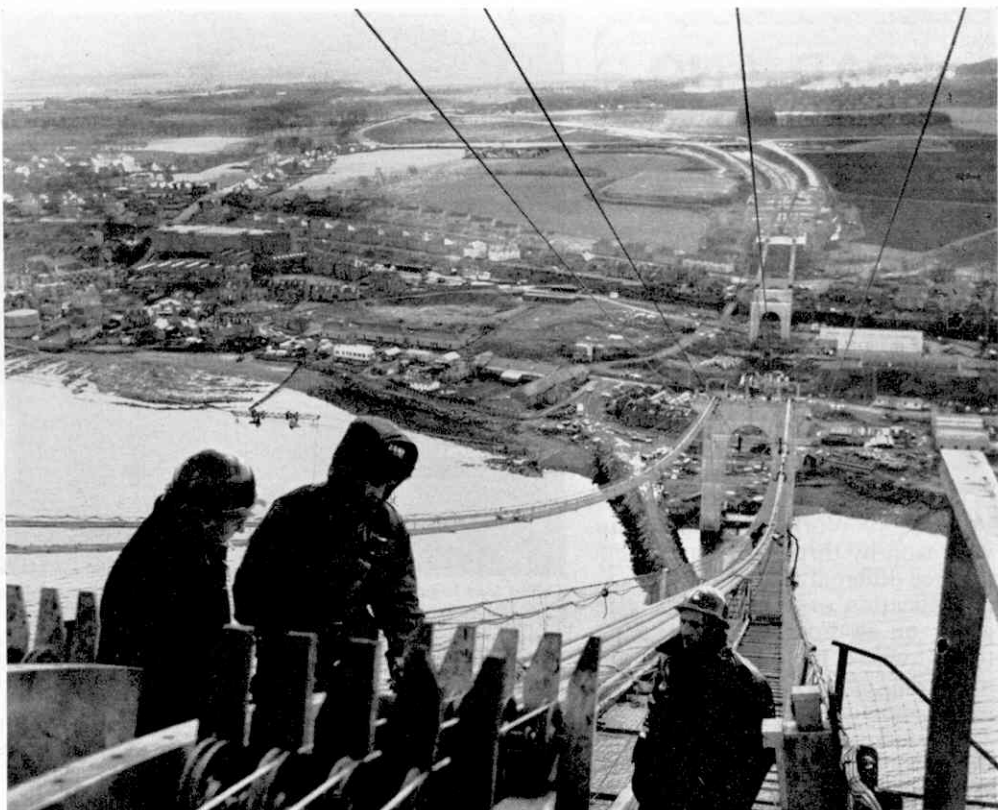
Top: High above Queensferry "spinners" are seen at work tensioning the cables 550 feet up. Left: In this unusual view the men at work on the bridge appear like human flies in the trough of the bridge's enormous span. Below: The business end of the bridge where the suspension cables are anchored, showing the world-famous railway bridge in the background. Pictures by courtesy of Keystone Press Agency Ltd.
