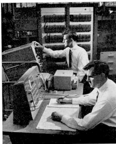
The KDN2 computer undergoing tests at the Kidsgrove Works of the English Electric Data Processing and Control Systems Division.
