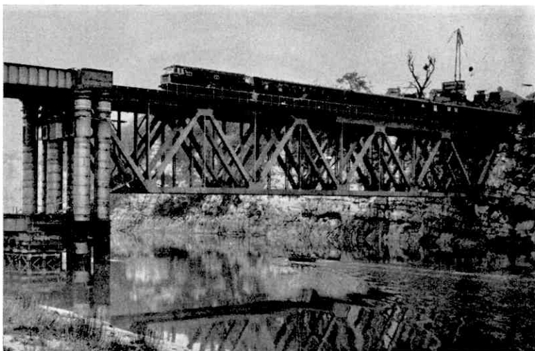
The bridge as it appears after rebuilding. The new spans are the pride of the railway engineers at Paddington.
