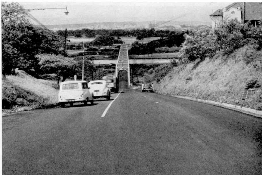
From South Africa comes this illustration of rubberised slurry seal surfacing on the approaches and deck of Athlone Bridge. Durban is in the distance.
