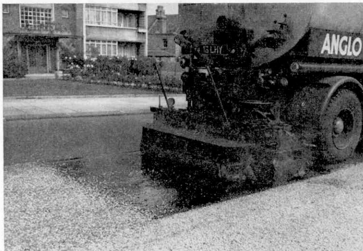
Rubberised bitumen being laid on Muswell Hill, North London.
