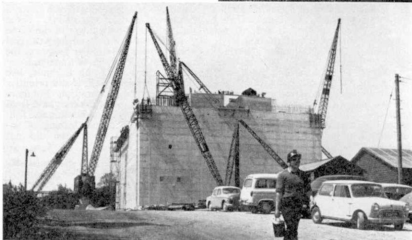
(Top) The Beachley Tower nearing completion. The roadway of the bridge will pass over the lower cross-piece of the tower. The Aust-Beachley Ferry, at present the only car-crossing south of Gloucester, can be seen on its journey across the river. (Centre) The giant Beachley anchorage nearing completion. (Below) A diagrammatic view of the new bridge, giving height and distances. Illustrations by the author.
