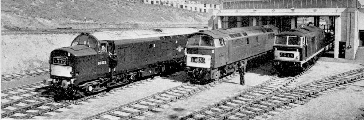
A view of the Landore Diesel Depot. Standing outside the shed can be seen three diesel locomotives—type 3 English Electric Co-Co, Western Enterprise class diesel 'Western Viscount', and type 3 Beyer Peacock (Hymek) B-B diesel locomotive.
