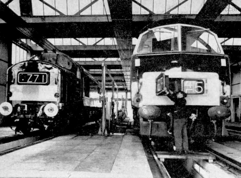
Inside the Landore Diesel Depot. The inspection pits for the locomotives can be clearly seen with modern lighting installed.
