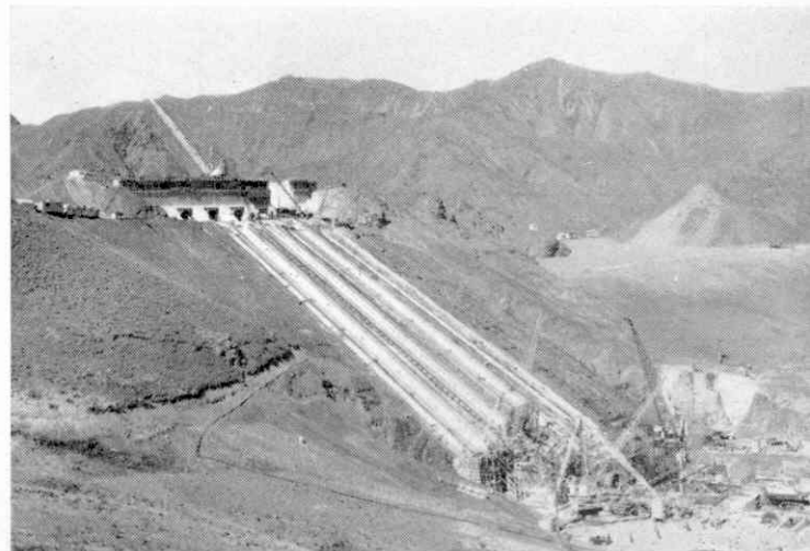
The penstock slope and power house construction.
