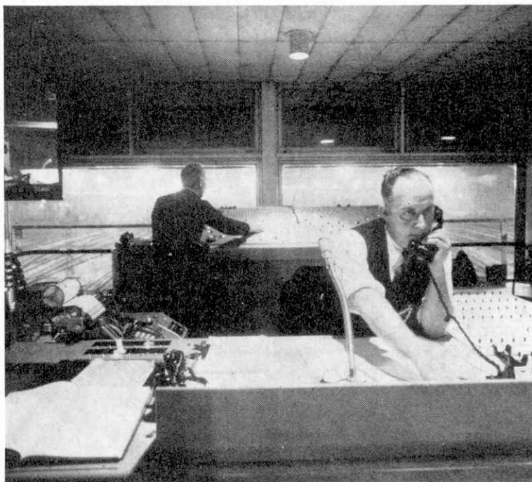
Night shift in the Tinsley marshalling yard control tower
