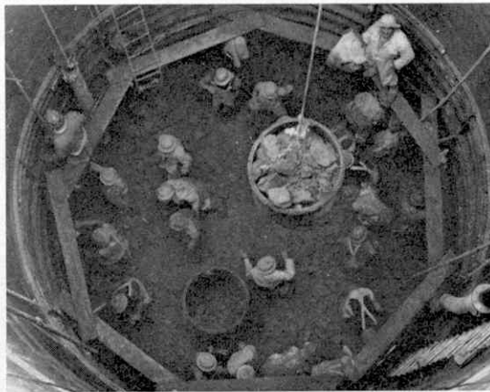
A shaft goes down on a new mine in South Africa. The faster the six shafts go down, the sooner do the investors get a return on the money they have laid out. The record for rapid shaft-sinking is held by Buffelsfontein, where 1,251 feet were sunk in March 1962.
