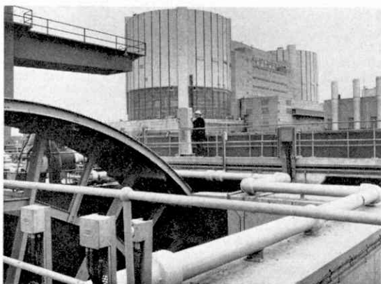
Below: A view taken from the C.W. system at the C.E.G.B.'s 600 MW Magnox power station built at Oldbury-on-Severn, Gloucestershire, showing, left to right, part of the cooling water system, the reactor block which contains the reactors and is linked by a common central services building, the central control building, the three gas turbine chimneys and the beginning of the turbine house. Started in 1960 the station was officially opened in June, 1969. Photo by courtesy of The Central Electricity Generating Board.
