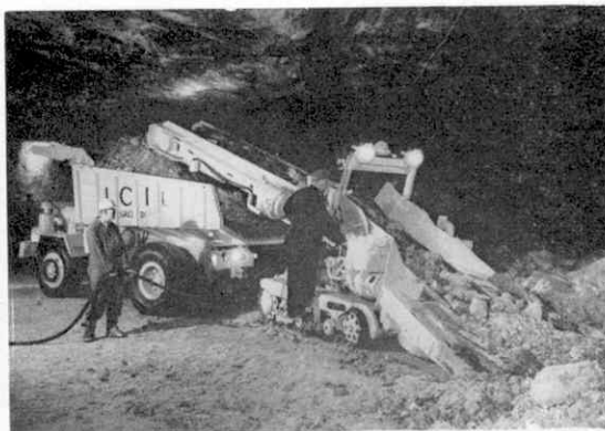
Loading rough rock salt at the working face. About 1,000 tons are blasted at each firing.
