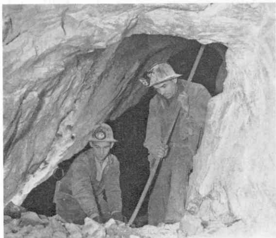
The scene after blasting operations at the Malagash mine, Nova Scotia, one of the largest mines in the Commonwealth. Miners are seen clearing a way through a mine passageway blocked by loose rock salt ore. Photograph: National Film Board.
