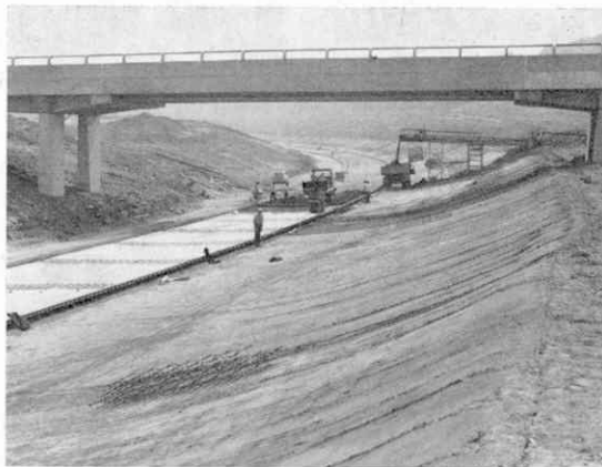
The banked two-mile circular test track is spanned by an access bridge strong enough to carry 40-ton loads. Vauxhall Motors Ltd.
