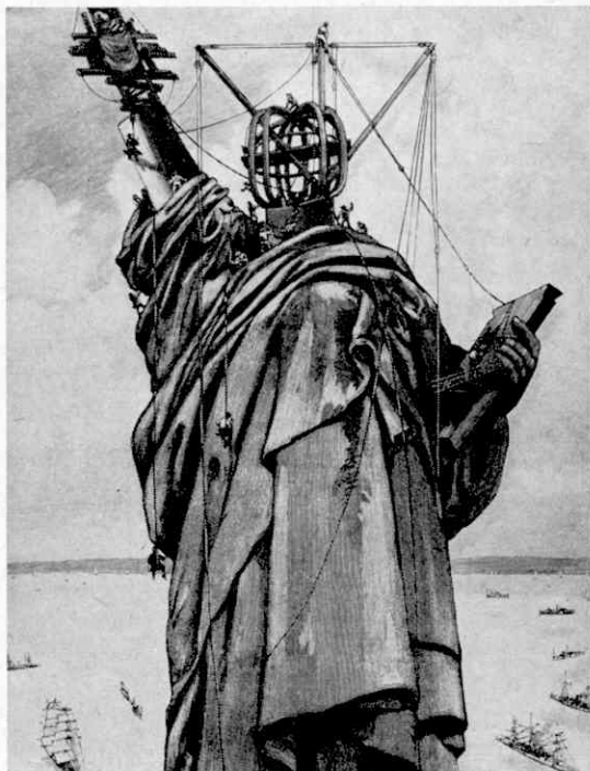
Rope-and tackle methods were used to build the Statue in America, after a trial erection in Paris.
