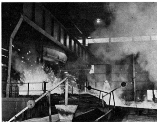
Top, one of the 3 L.D. vessels shown during blowing cycle. This vessel produces approx. 130 tons of steel every 45 minutes
