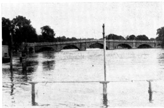
The bridge over the Thames at Richmond, built in 1773, just before the first iron bridge. The width was doubled in the 1930s.
