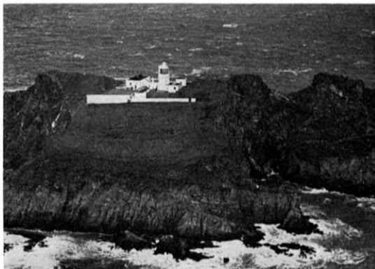
Approaching Lundy South. The landing pad for cargo and winches is on the little hill to the right of the lighthouse.
