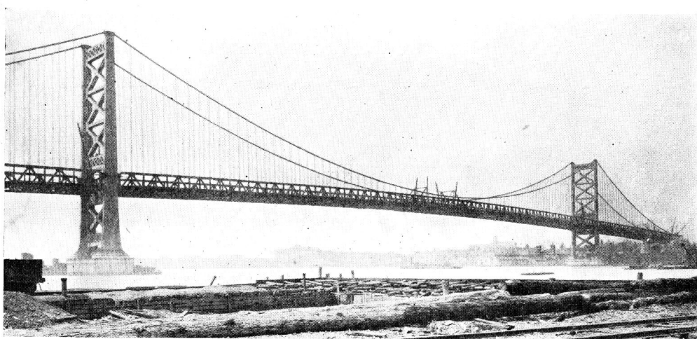
The Delaware River Bridge in Course of Construction
